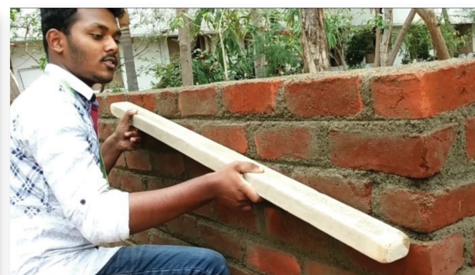
BRICK WORK CONSTRUCTION
